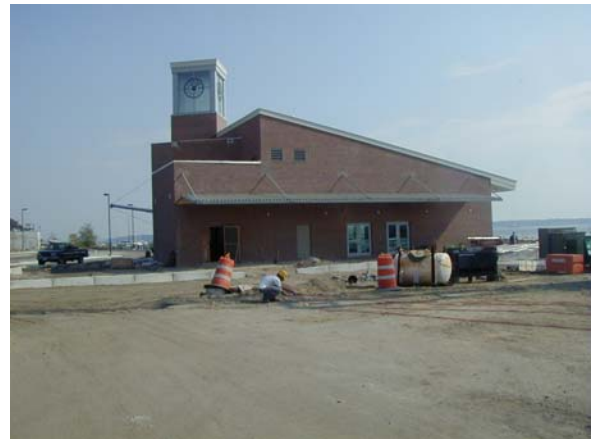
Receiving Station under construction at Ocean Gateway site
