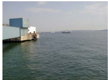
Future site of Megaberth
