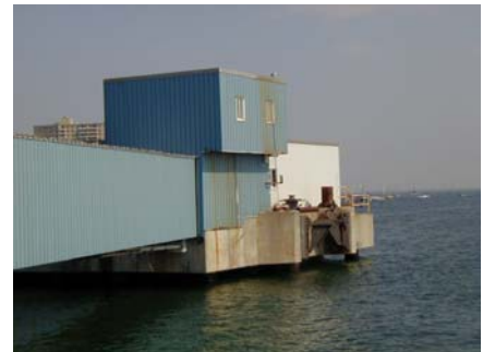
Mooring Platform No. 1
