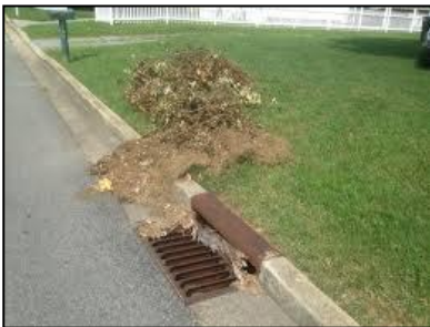
STORM DRAIN & ESPLANADE
