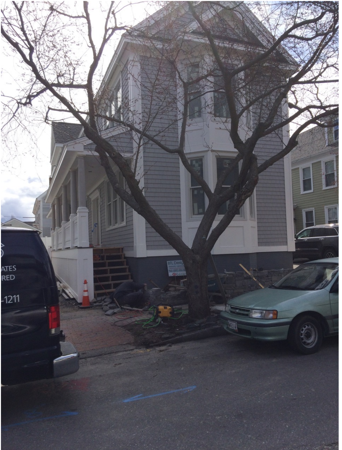
HOWARD STREET NEW CONSTRUCTION
