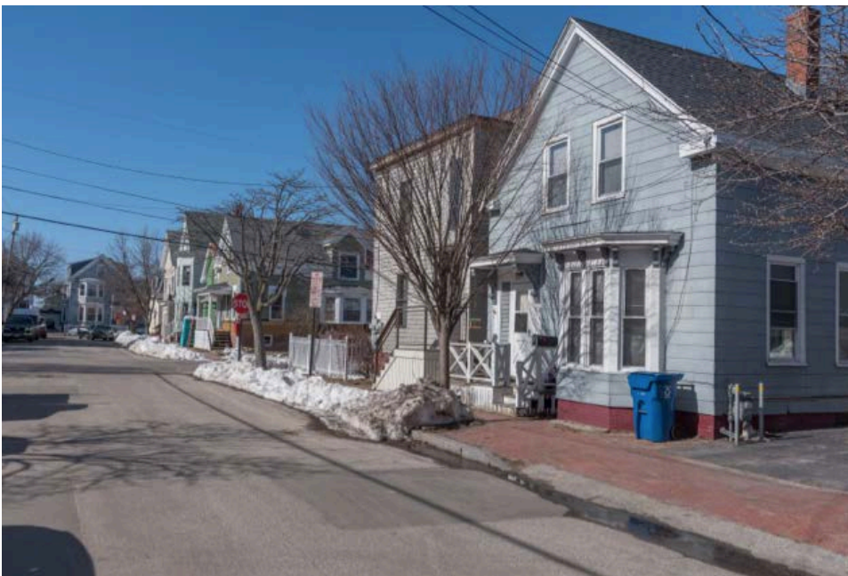
The second and third blocks of Merrill Street: small residential, New England character
